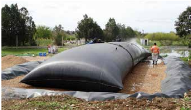
Fig.1 Geotextile tubes used for capturing and further dewatering sludge for disposal in solid form
