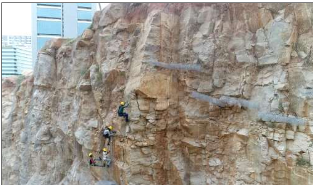
Fig. 5 : Installation of RockFall nets of Double Twist Mesh on the slope.
