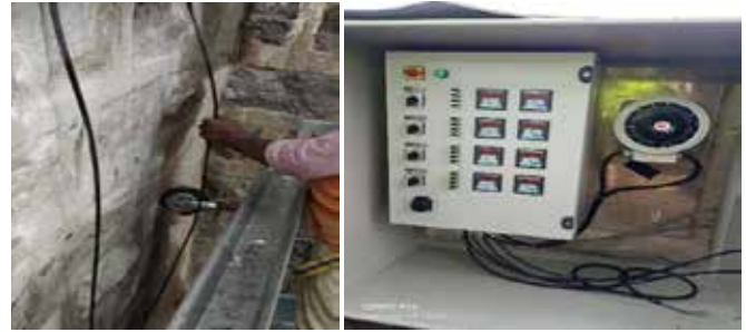
Fig. 11 : Installation of Optical fiber cable and the control units
