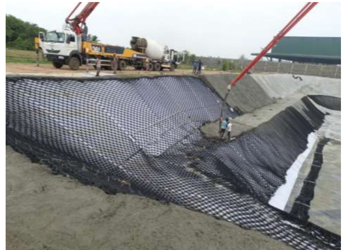
Fig. 7 : Filling of concrete on the installed geocell layer
