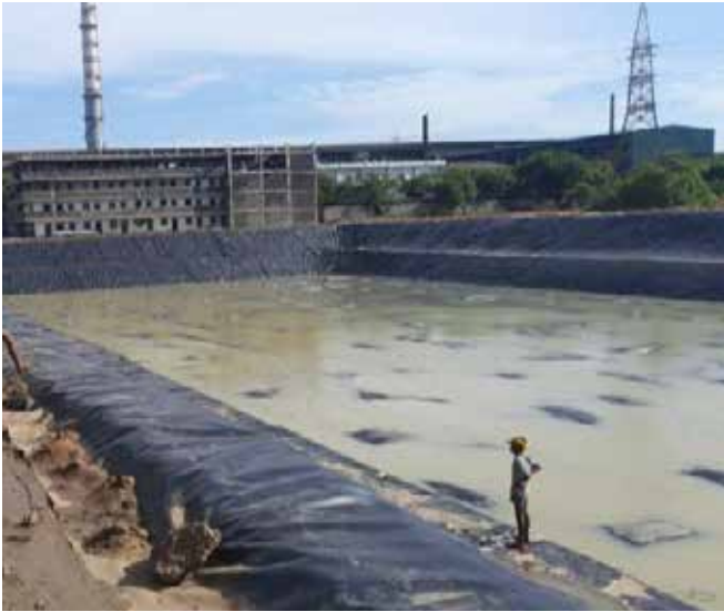
Fig. 5 : Installed geomembrane layer on the surface of reservoir
