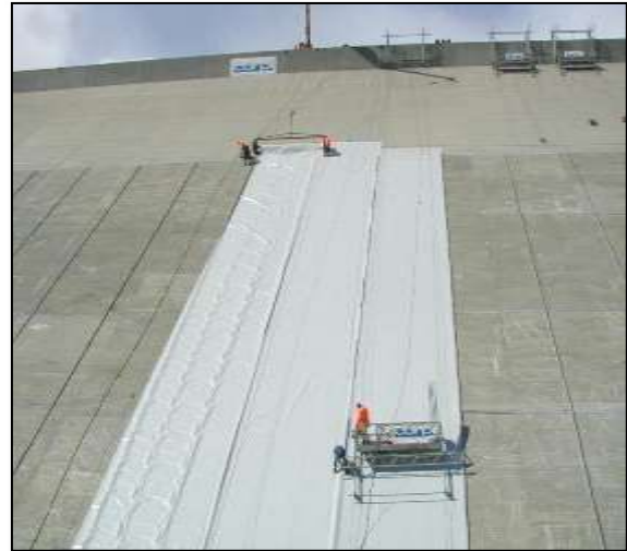
Picture 4: Effect of the Carpi tensioning profile system. (Left) Winscar dam (UK, 2001) and (Right) Midtbotvatn dam (Norway, 2004).
