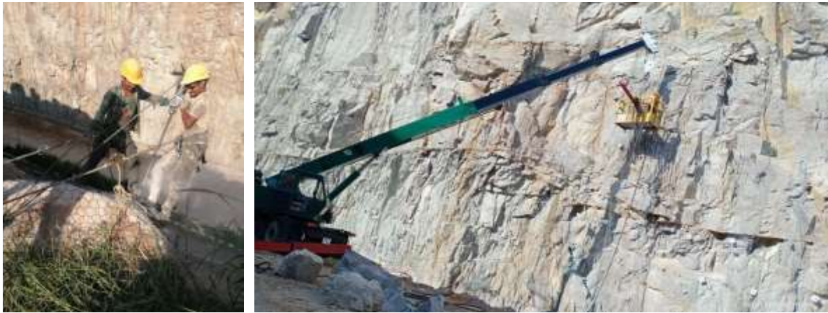
Fig. 4 : Installation of Anchors on the slope.
