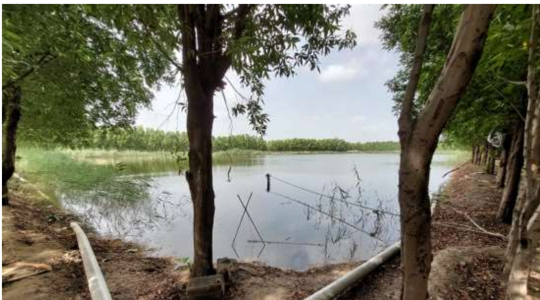
Fig. 1 : Industrial water pond with 1.5 mm HDPE Megaliner
