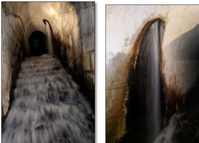
Picture 3 : Water gushing from the 2 shafts near the spillway
