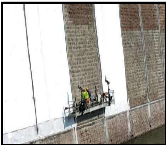
Fig. 7 : Thick 2000 gsm geotextile installed
