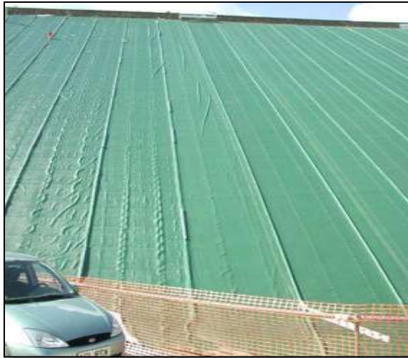
Picture 4: Effect of the Carpi tensioning profile system. (Left) Winscar dam (UK, 2001) and (Right) Midtbotvatn dam (Norway, 2004).
