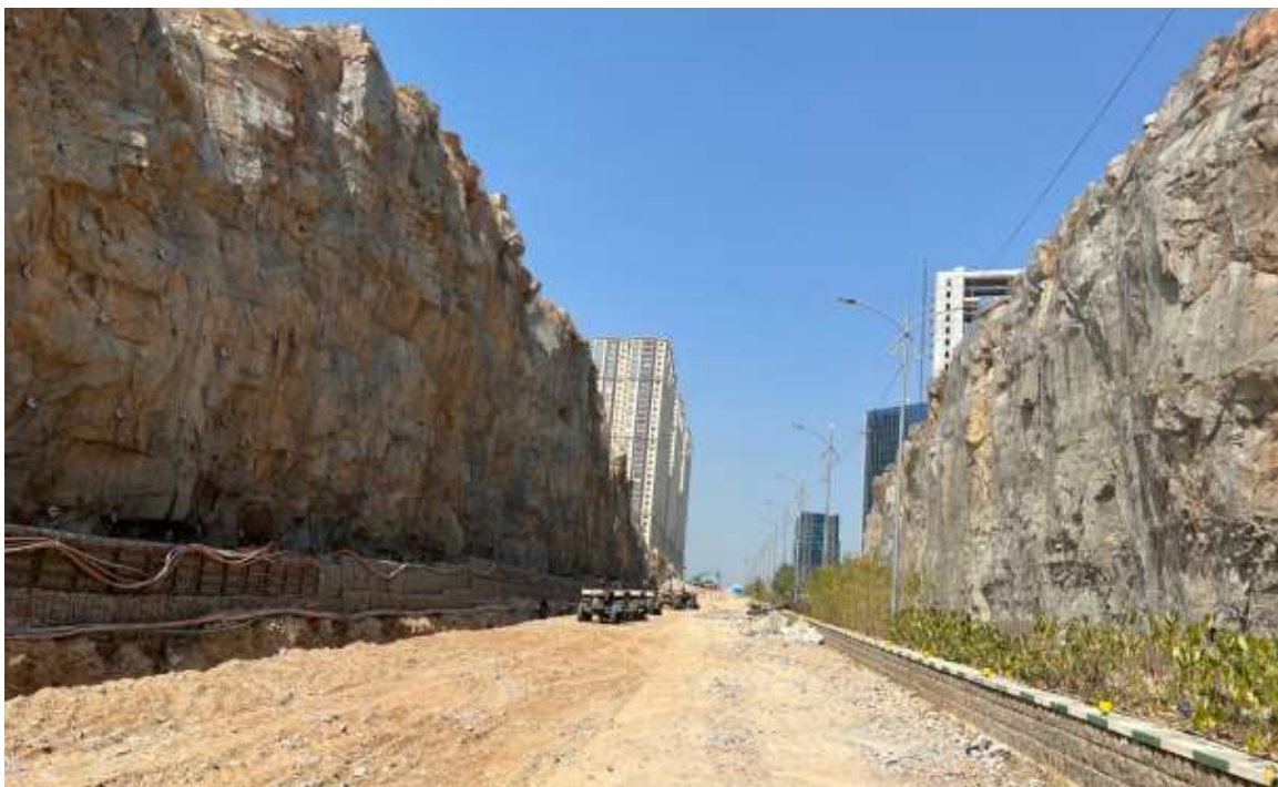
Fig. 7 : View of the completed work.
