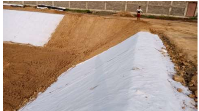
Fig. 4 : First later of geotextile laid over the prepared surface
