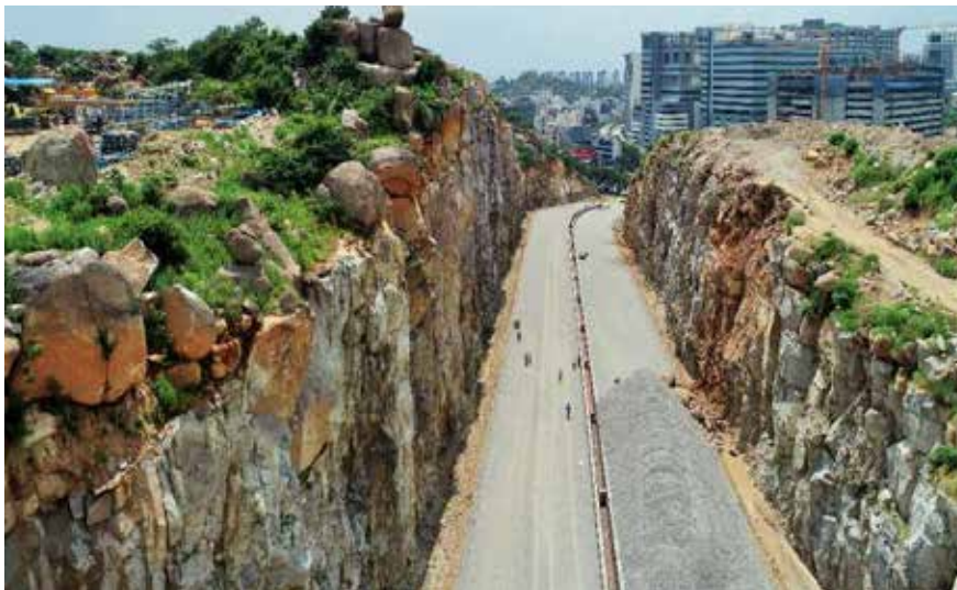
Fig. 1 : Site photo prior to the protection works showing the loose rocks on the slope and top.
