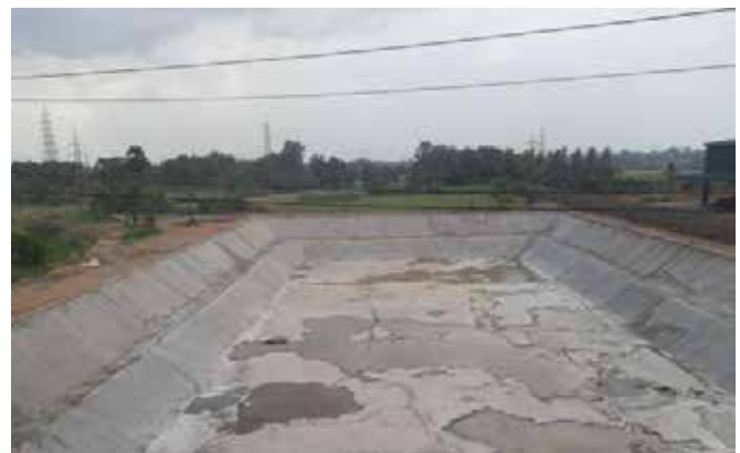
Fig. 8 : Finished raw water reservoir lining
