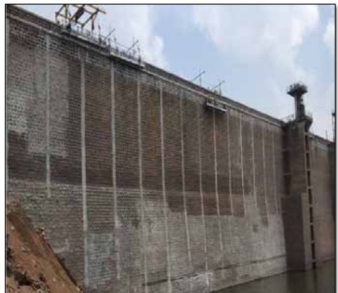
Fig. 6 : Preparation of mortar strips for placement of vertical anchorages
