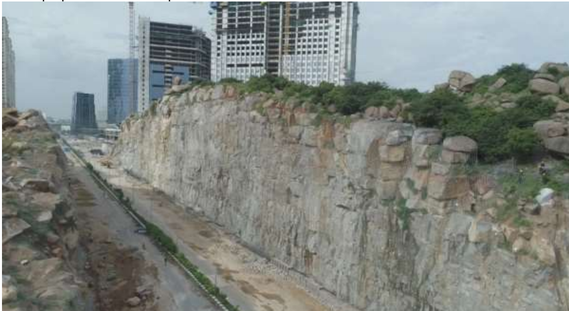
Fig. 6 : View of the installed nets on the slope.
