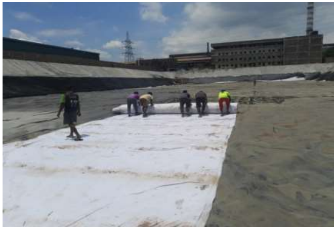
Fig. 6 : Installation of second layer of geotextile on the top of geomembrane
