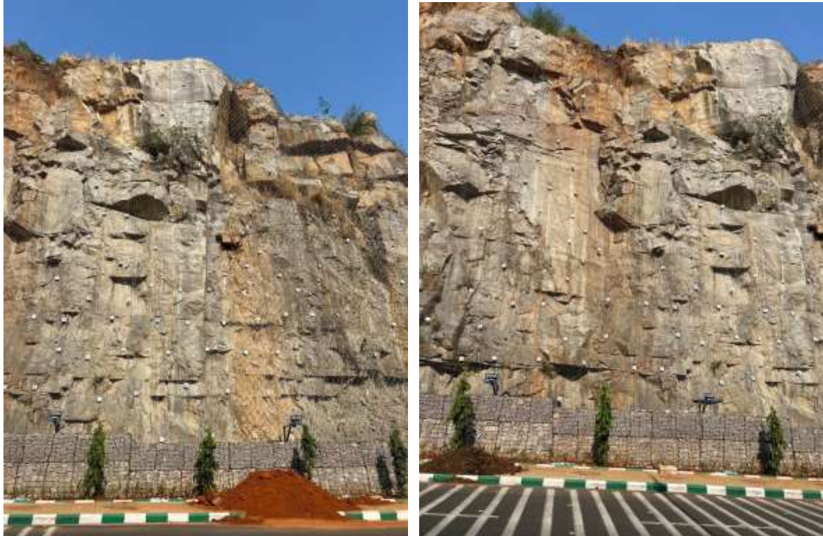
Fig. 8 : Site photos after one rain with stones entrapped in the nets
