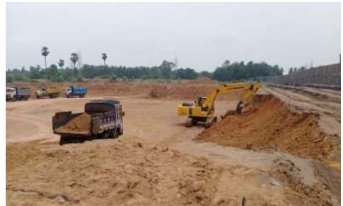
Fig. 3 : Excavation to create a reservoir
