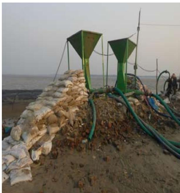
**Fig. 6 :** Slurry mixing tank used at the project site
