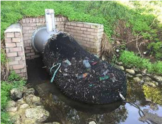
A net safely captures waste plastic from a drain
