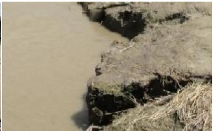
Fig. 5 : Vulnerable bank condition before undertaking anti-erosion works
