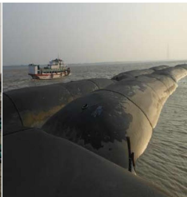
**Fig. 7 :** Installation of bottom tier geotextile tubes
