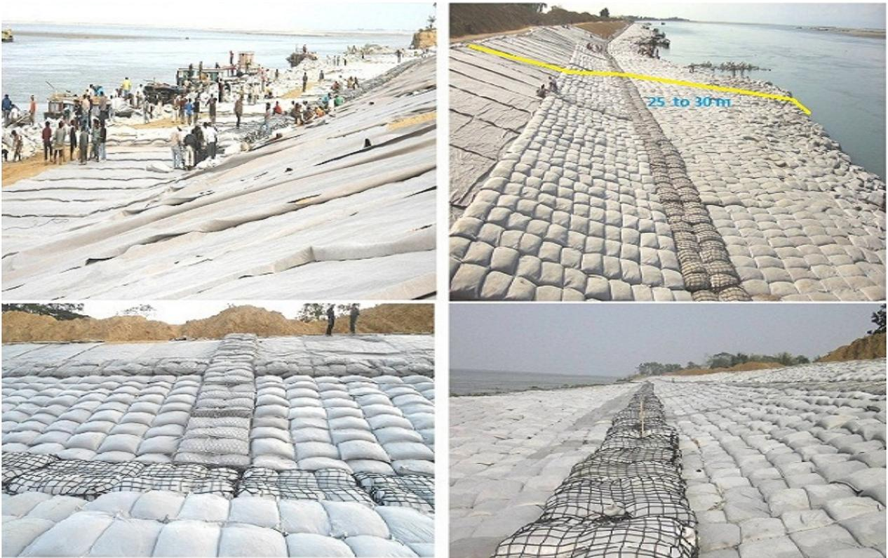
**Fig. 5 :** Placement of filter media, Geobags & PP Gabions
