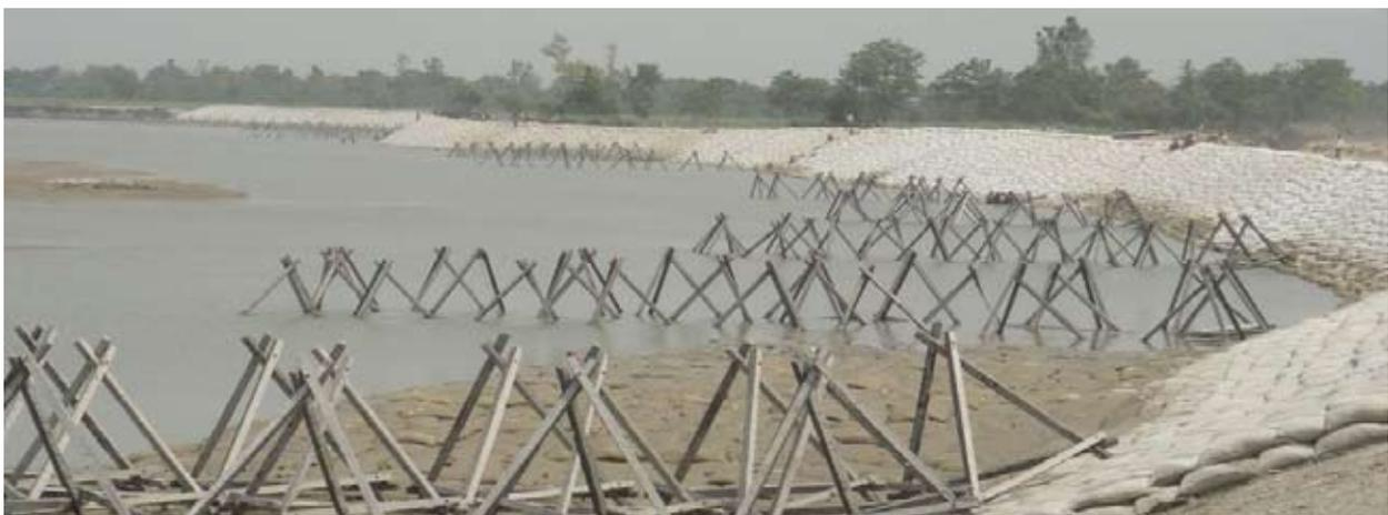
Fig. 7 : Protection work using geotextile bags and porcupine spurs
