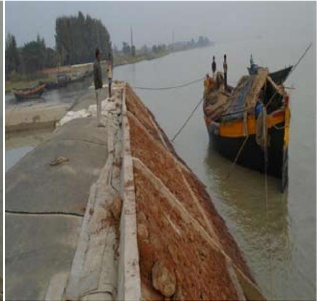
**Fig. 9 :** Boulders placement on the geotextile tube
