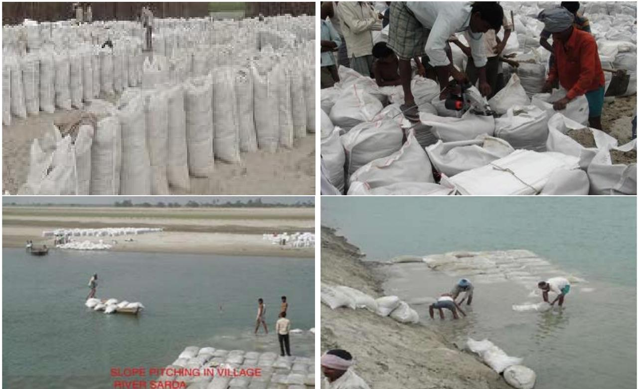
Fig. 8 : Filling, transportation and installation of Geotextile bags [8]
