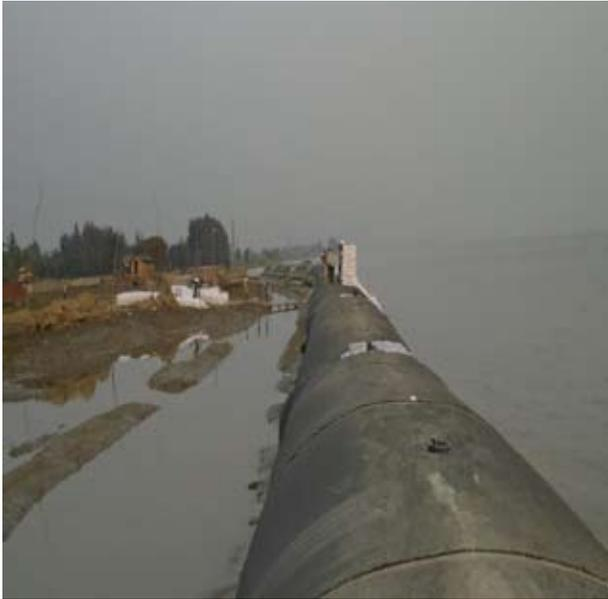
**Fig. 8 :** Installation of second tier geotextile tube
