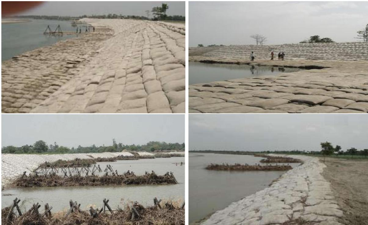
Fig. 11 : Implementation of geotextile bags in revetment and launching apron
